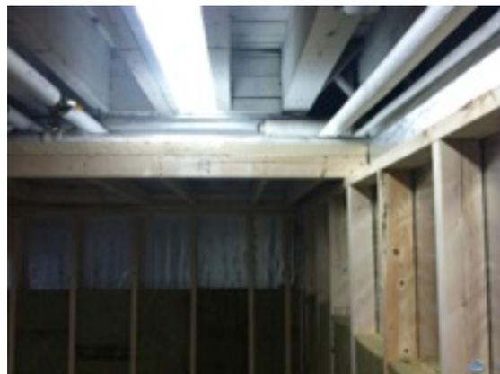
If you notice in the above photos, we laid the 2" insulation all the way down the outside of the floor, then built the wall frame on the floor itself, so we would not have any leaking of cold air. We also cocked heavily around these areas to make it airtight.
