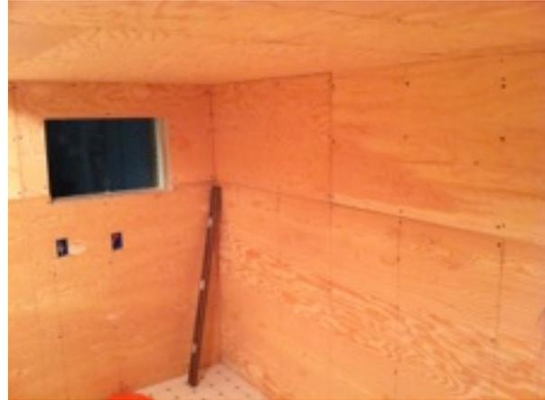
The photo above shows the layers of insulation, the interior plywood layer, and the opening for the air conditioner.
