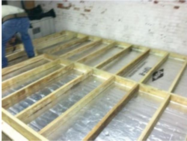
Once that was complete, we laid in Roxul, which is a high-end house insulation, 4" thick. Roxul is not affected by moisture or cold, however it certainly is more expensive than traditional fiberglass insulation. It has an R-value of 16.
