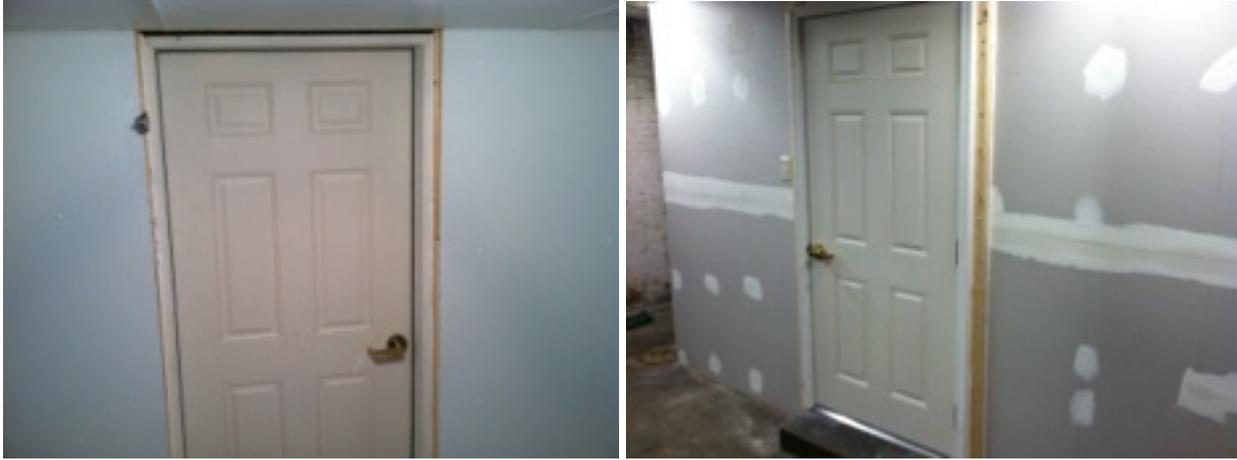
To finish the unit we sheetrocked the outside of the box. This unit is in a basement so we are not too concerned about the outside finishes.
