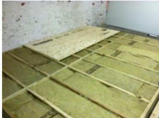
We were very careful to make sure the insulation and box were extremely tight and sealed, then we added 3/4 inch flooring plywood over the frame.
