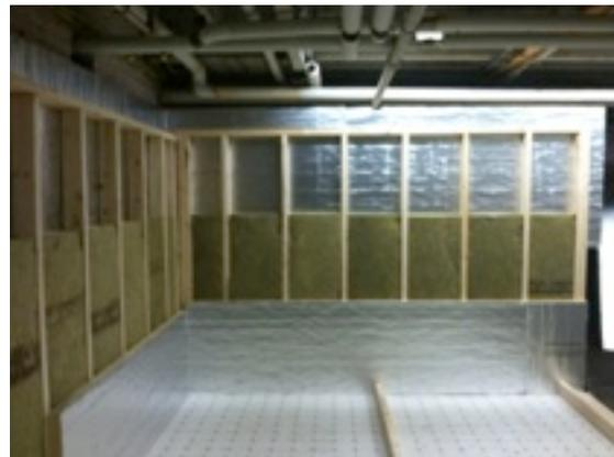
The ceiling was the biggest challenge, as you can see from the above photo. We have lots of pipes in the basement, including sprinklers. The back of the cooler's inside ceiling height is 5'11", and the front of the cooler is 6'3". We built two different ceiling frames and stepped them so we could get as much height as possible. We also built a hatch just in case the sprinkler heads or water shut offs had to be accessed in the future.
