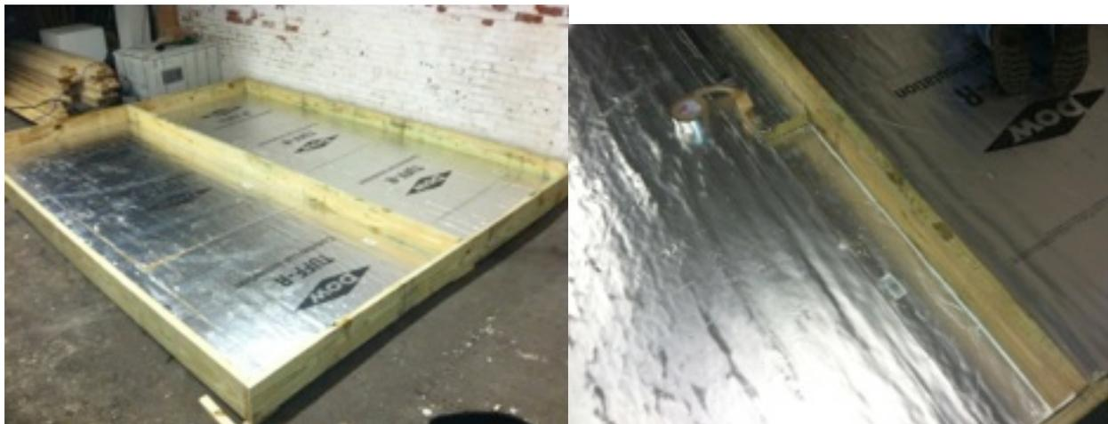
We then built a frame out of pressure treated 2x4s inside the floor box.
